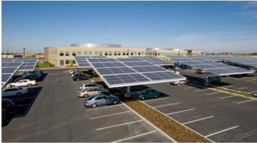
Figure 1: Example of a Dual Use Solar Panel Installations
