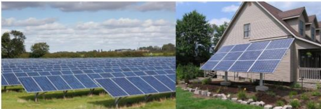
Figure 3: Examples of Ground-Mounted Solar Panel Installations
